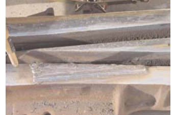
Completed Weld on a Frog
