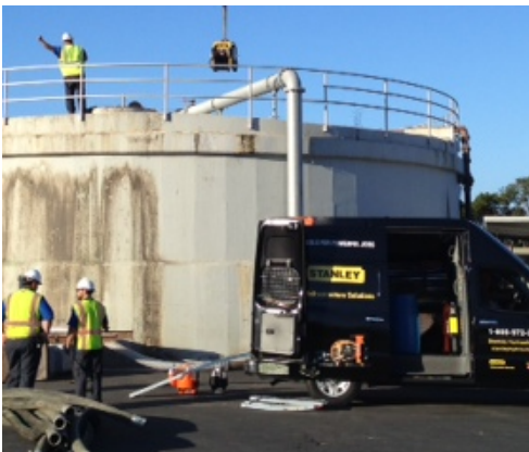
HP28 Power Unit being lowered onto tank roof
