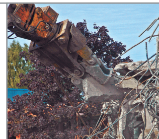
UPX 950 WITH CONCRETE PULVERIZER JAWS
